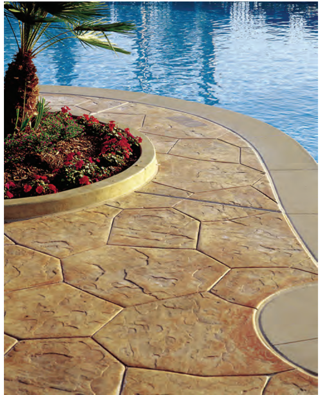
Fig. 1.1b—Concrete slab enhances design aesthetic with mimic of stone slab (courtesy of L. M. Scofield Company).
