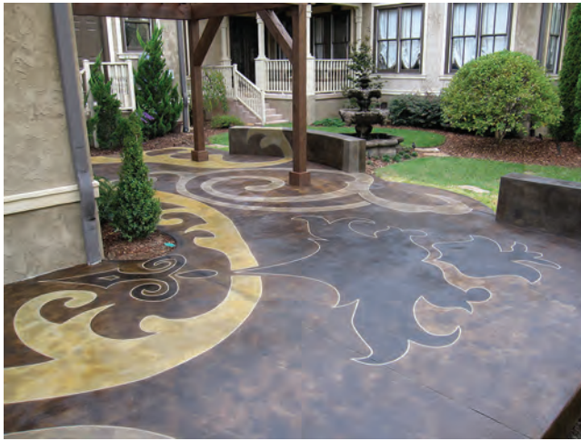
Fig. 1.2—Cast-in-place decorative concrete combining treatments during and post placement to achieve aesthetic effects (courtesy of Concrete Mystique Engraving).
