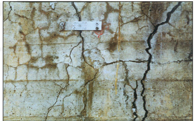
Fig. 2—Monitoring changes in crack width.
