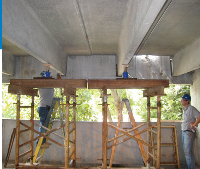
Responsibility in Repair Construction
